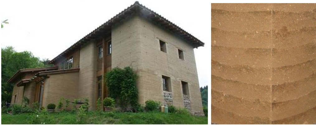
Fig. 1. Left: a rammed earth house in France. Right: a rammed earth sample.
